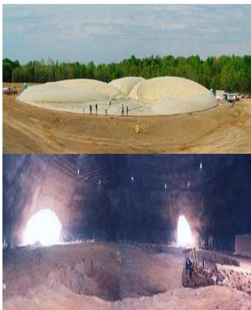
Fig:3.1.3 Shotcrete applied to inside of inflated fabric form
